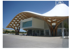
Fig. 7. Canopy, Centre Georges Pompidou, Metz (from: author)
