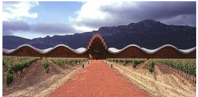
Fig. 23. Roof Design of Bodegas Ysios Winery
