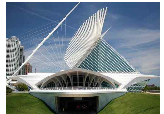
Fig. 13. New Building of the Milwaukee Art Museum
