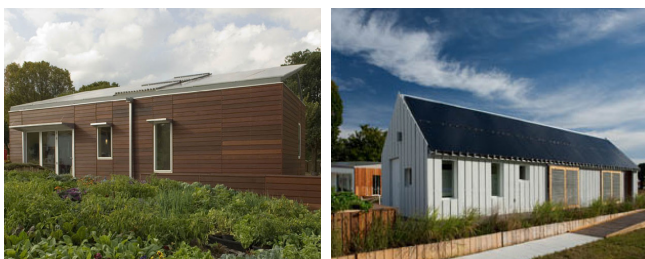
Fig. 3. Solar Energy Generation System with PV Cell, Team Cornell University (Left), Gable Roof with BIPV System, Team University of Illinois, Urbana-Champaign (Right)
