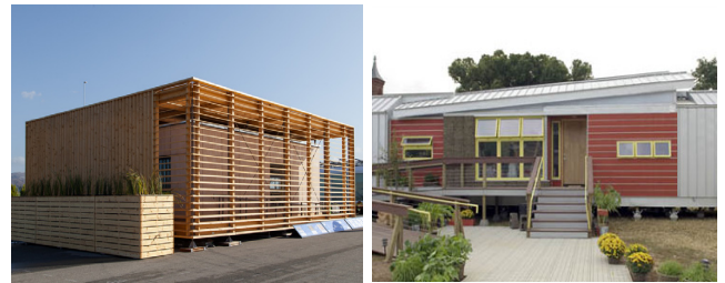
Fig. 4. Double Building Envelope with Wood Materials, Team Czech Technical University (Left), Bio-SIPS Insulation Materials, Team University of Illinois, Urbana-Champaign (Right)
