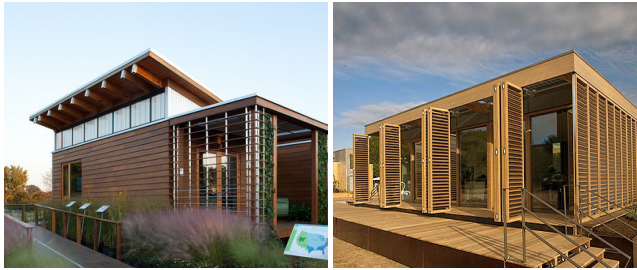
Fig. 2. Butterfly Roof for Daylighting and Ventilation, Team University of Maryland (Left), Flexible Shading System with Oak, Team Technische Universität Darmstadt (Right)
