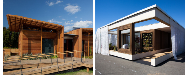
Fig. 6. Butterfly Roof and Shading Device, Team Victoria University of Technology (Left), Fabric Curtain at Exterior Space, Team Vienna University of Technology (Right)
