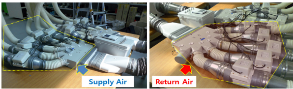
Fig 5. Air distributor of supply and return line
