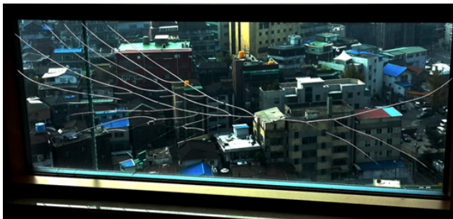
Fig 2. glazing breakage due to thermal expansion
