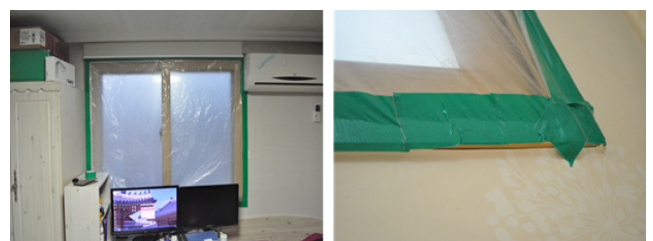
Fig. 2 Sealing of windows
