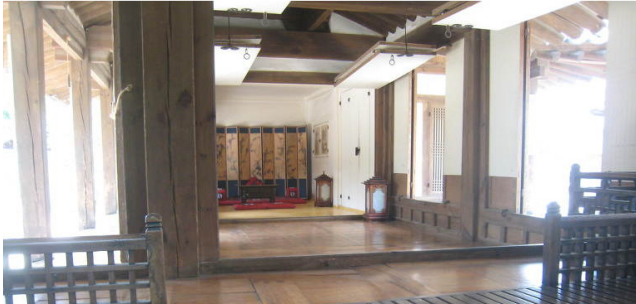
<Figure 3> Lift-open structure door-wall in the room of Yoon Taek-Young, Haepoong Buwungun
