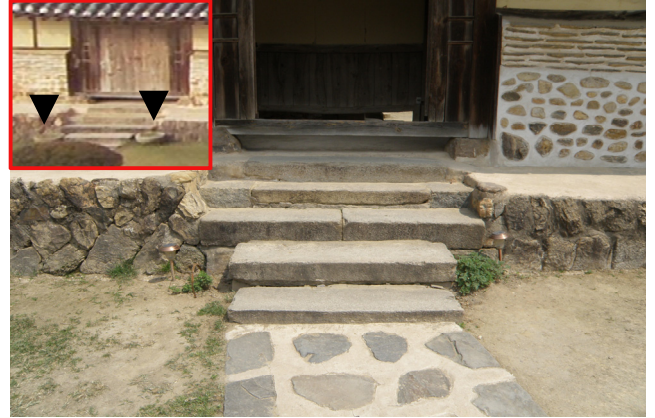
Fig 11. Lower Lintel and Stone Step A stone mortar was located at the old picture in red line.
