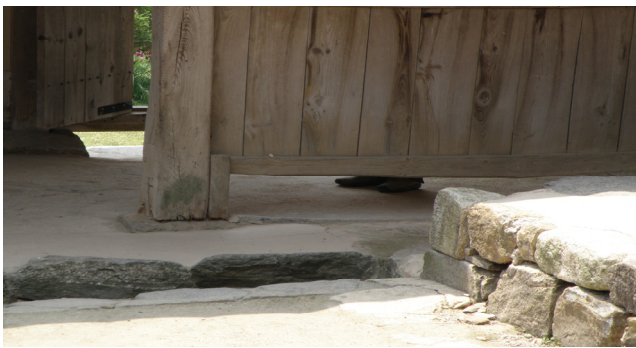
Fig 10. A Fake Wall inside the Main Gate for Watching Visitor
