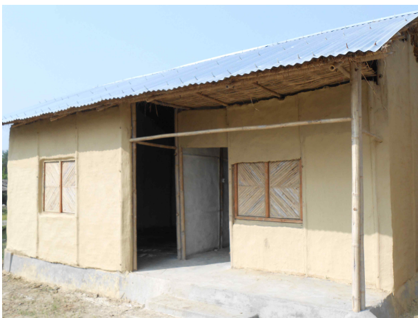
Fig. 7. Double panel bamboo house before installation of doors
