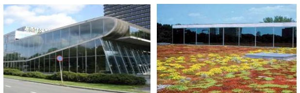
Figure1. Side and green roof view of Educatorium 5)
