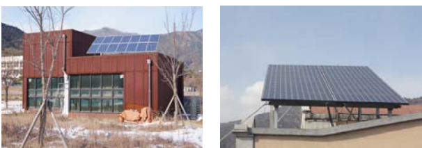
Fig. 16. A typical PV installation on Flat roof in domestic
